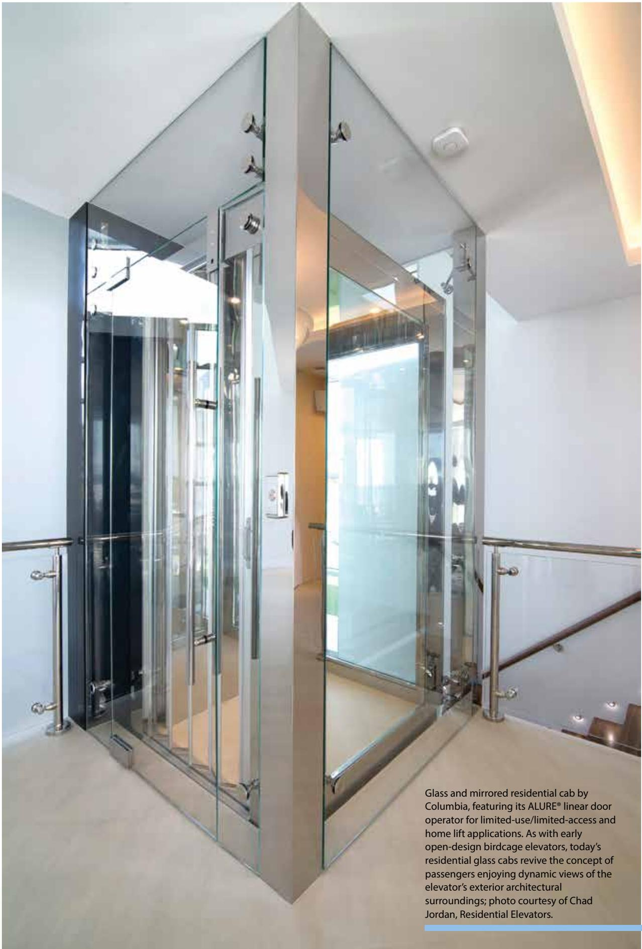
Glass and mirrored residential cab by Columbia, featuring its ALURE® linear door operator for limited-use/limited-access and home lift applications. As with early open-design birdcage elevators, today's residential glass cabs revive the concept of passengers enjoying dynamic views of the elevator's exterior architectural surroundings; photo courtesy of Chad Jordan, Residential Elevators.
