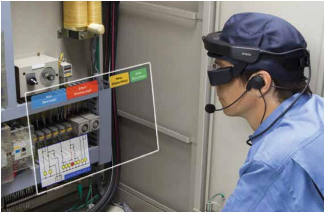
Elevator equipment operation in the field can be managed using AR technology on a headset. Seen here is a technician monitoring faults using the elevator controller's wiring diagram.
