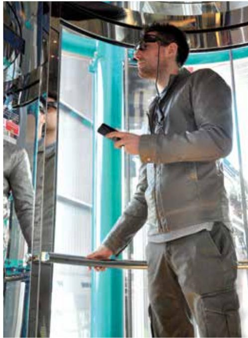
A service technician is (l-r) on a car top, wearing a head-mounted display running diagnostics to troubleshoot door-operator performance and, inside a car, adjusting door parameters to set open and close times and performance modes such as “Night Shift,” “Rush Hours,” etc.
